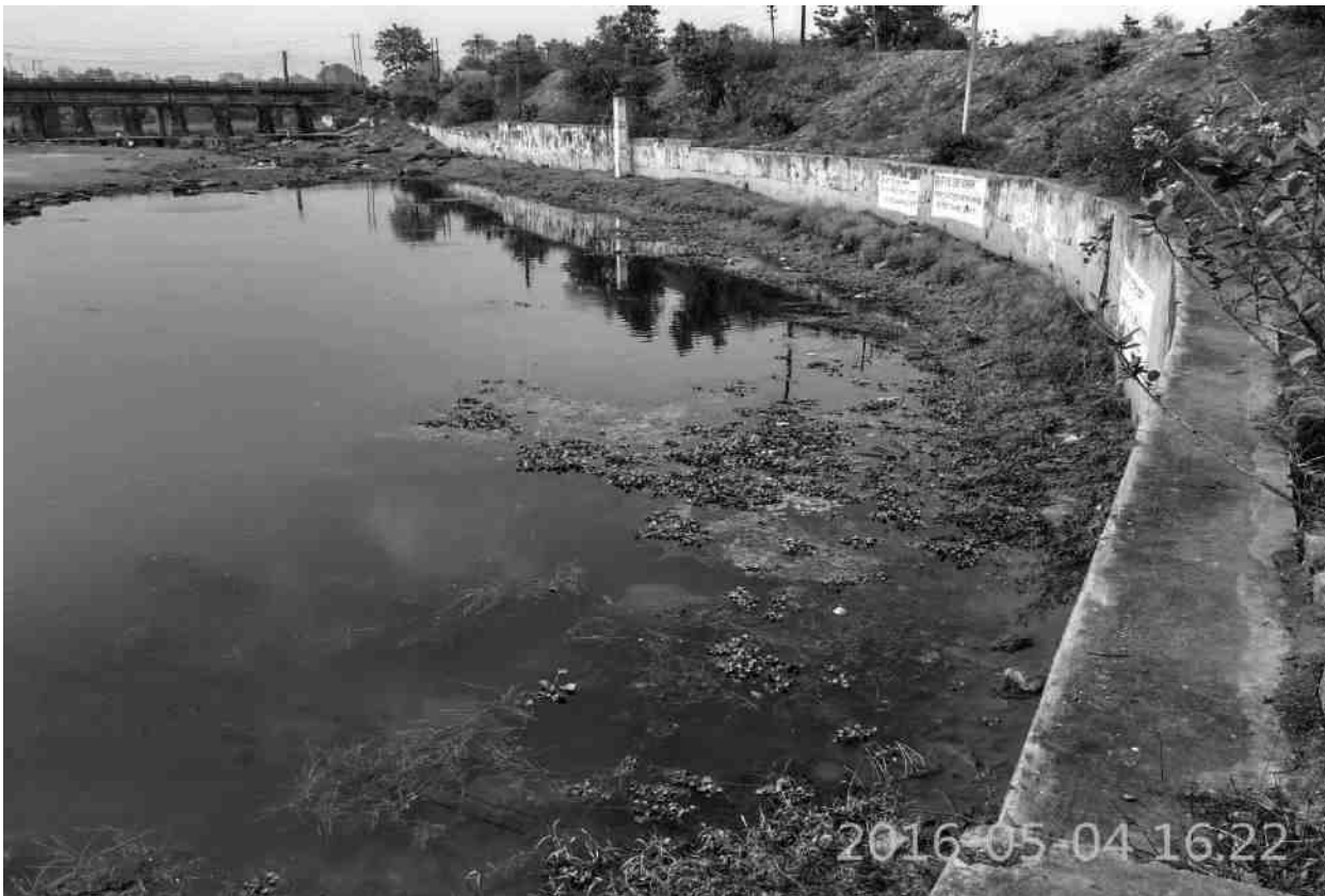
Toe wall and Embankment at Cluster IV
