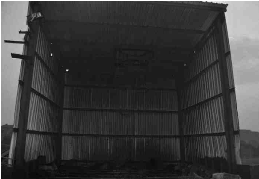
Water Arrangement at CHP Hooper
